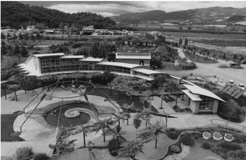
FIGURE 23. Showroom, site and surroundings
